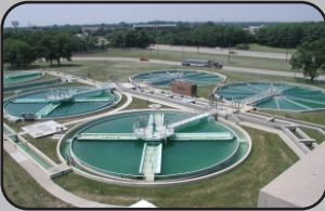
Water Treatment & Filtration Plants
